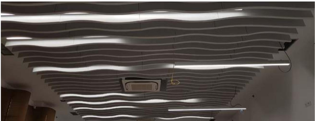
The acoustic baffles **ALPHA**coustic-Sine can be produced in different shapes, dimensions and thickness upon request.
